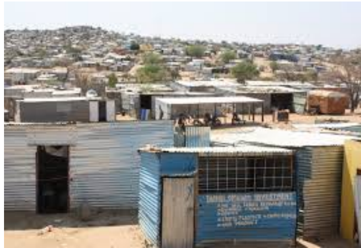
Typical informal settlement housing structure in Namibia made out of corrugated sink
